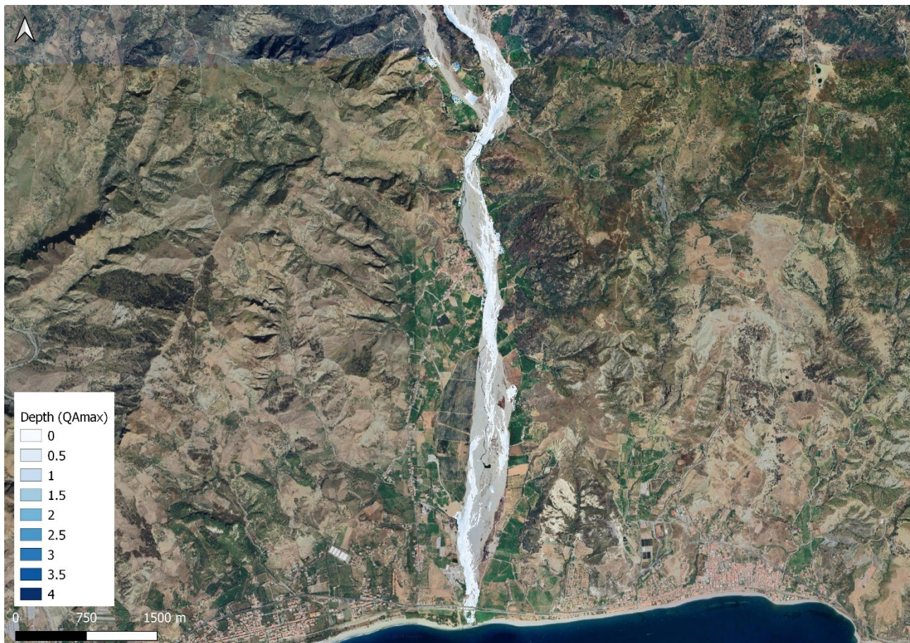
Figure 6. Floodable areas downstream of the Menta dam related to QAmox.
