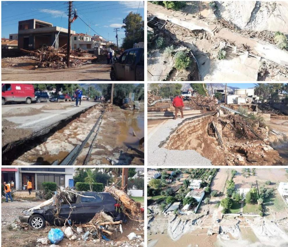
**Figure 3.** Damages by the flood of 2019 to infrastructure, road networks, and the coastline of the Kineta area [55–57].
