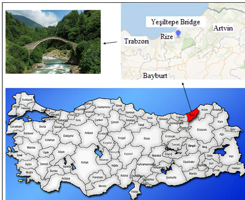
Figure 1. Location and appearance of the bridge.
