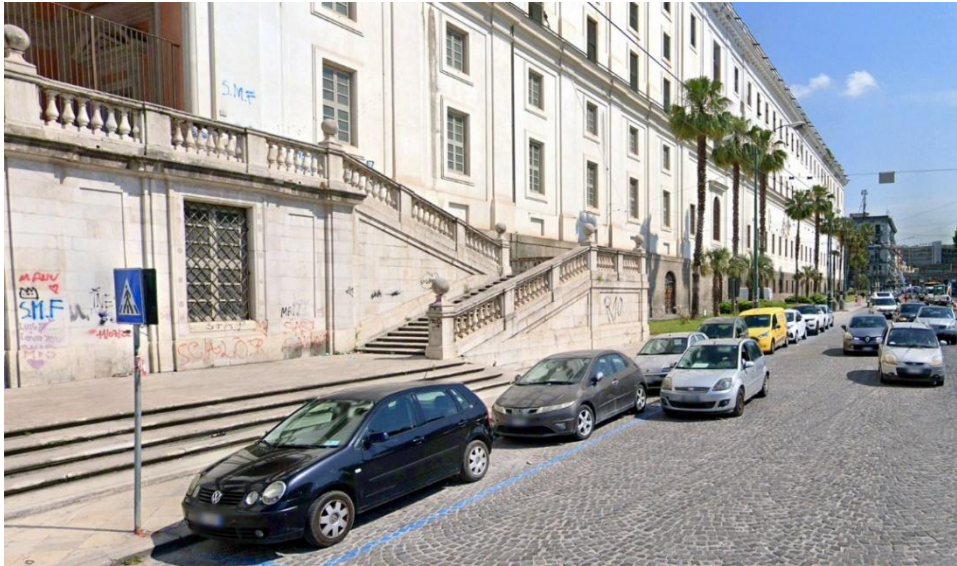
Figure 5. Naples: Real Albergo dei Poveri or Palazzo Fuga, current view. The building suffered severe damage in the infirmary, part of the refectory and some of the rooms on the first and second floors.
