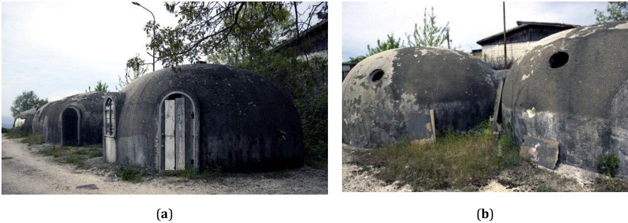
Figure 9. San Potito Ultra (Avellino province) temporary housing consisting of thermo-igloos, which were dismantled only a few years ago (Photo by Sabina Porfido, [47]). (a) Examples of temporary accommodations; (b) Detail of the thermo-igloo of San Potito Ultra (Avellino).
