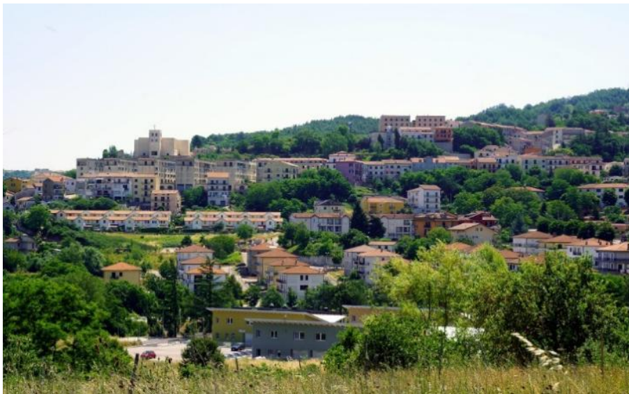
Figure 22. Teora (Avellino province) Rebuild the village according to construction criteria that favor the use of reinforced concrete (Photo by Porfido & Spiga 2022).
