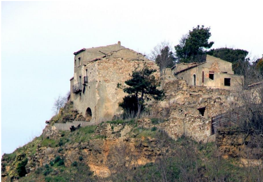
Figure 15. Conza della Campania (Avellino province). Examples of very poor constructions consisting of rubble stone with little mortar were very common at the time of the 1980 earthquake throughout the historic centers of the Campano-Lucano Apennines (Photo by Porfido & Spiga 2021).
