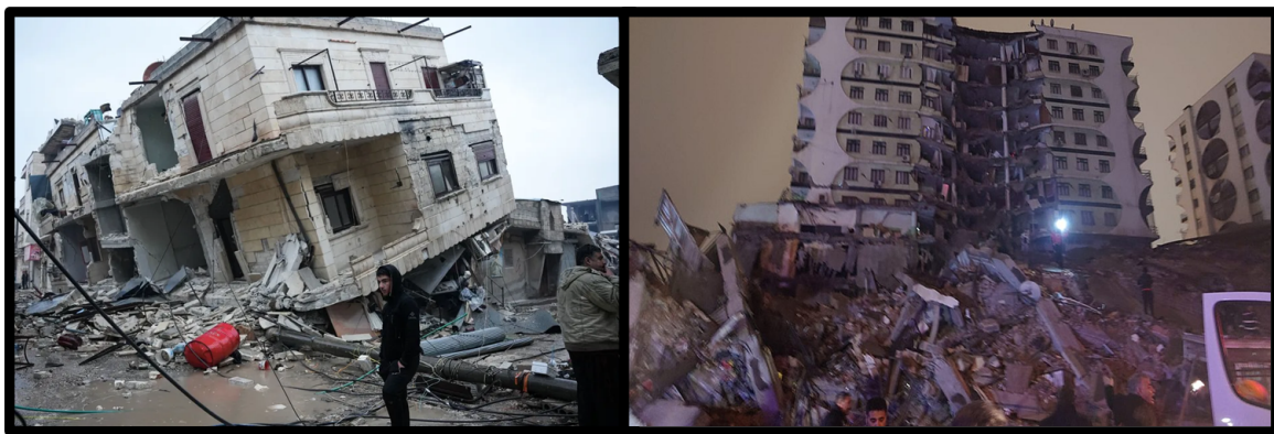
Figure 3. Illustration of building damage [16,17].
