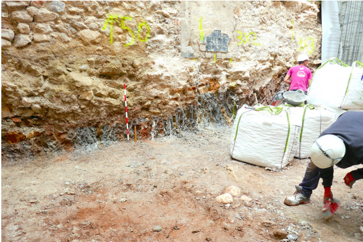
Figure 2. Southwestern part of the excavation site showing middle Miocene compacted lutites directly below the foundations of the Aguado alley wall. The bar (1 m) gives the scale. View from the southeast.
