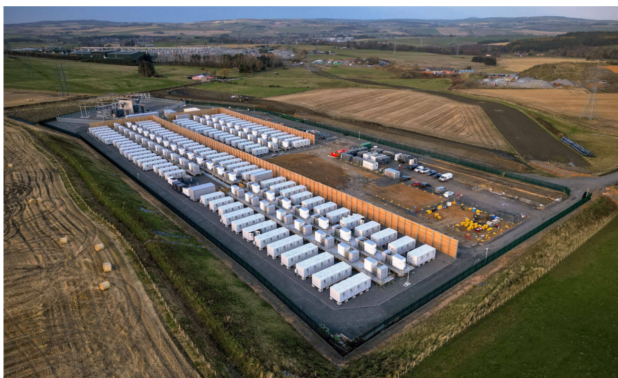
Figure 4. Offshore Wind Electricity Feeding Directly into Containerised Lithium Batteries by Zenobe, Europe's Biggest Battery at Blackhillock, Scotland [15,16] .
