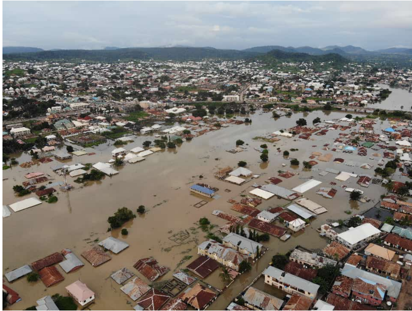
Figure 1. Submerged Houses in Kogi State Flooding.
